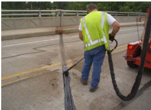
2014 Crack Sealing Program
