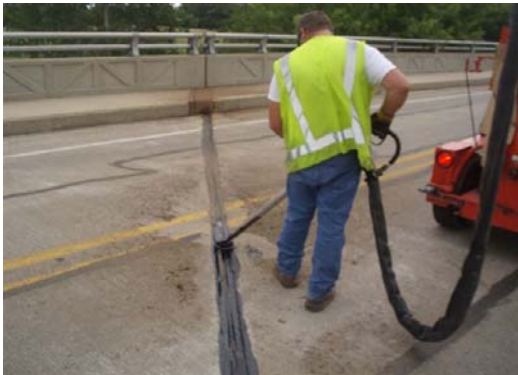
2015 Crack Sealing Program
