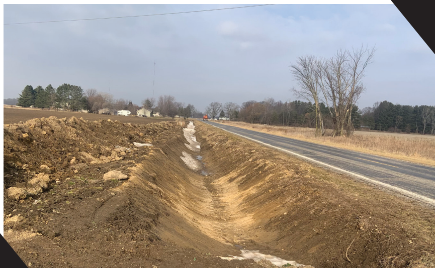
Ditching / Drainage Maintenance
