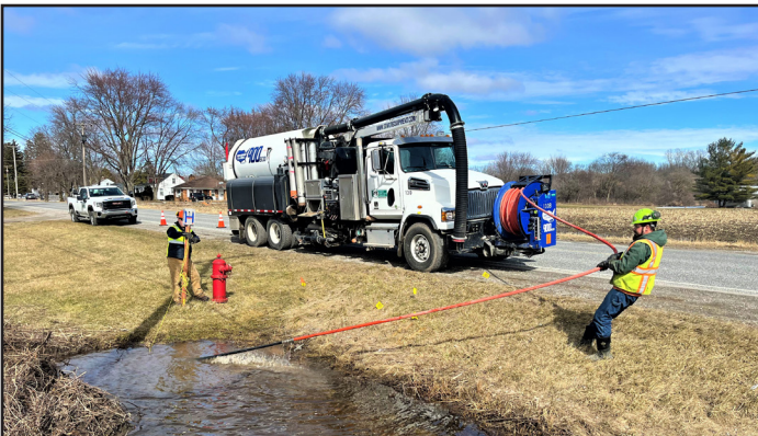
Sheridan Rd at Young Rd - Spaulding Twp Tile Jetting (Hydro Excavating)
