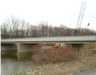
Fort Rd. Bridge Reconstruction
