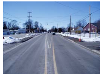
Shattuck Rd. Paving Project
