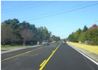
Brockway Rd. Paving Project
