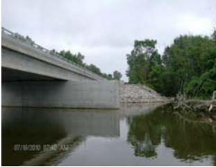
Center Road Bridge Reconstruction
