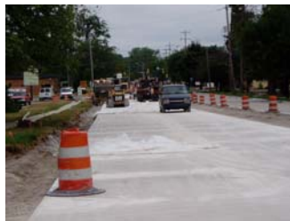
Dixie Hwy. Reconstruction
