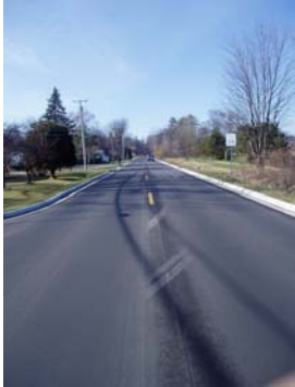
State Street Paving Project
