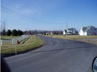
N. Thomas Road Paving Project
