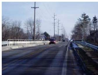
Freeland over the Tittabawassee River—Bridge Reconstruction
