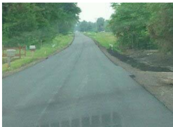
Ferden Road Paving Project
