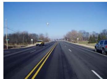
Dixie Highway over the Cass River—Bridge Reconstruction
