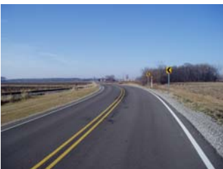
Wadsworth Road Paving Project
