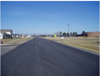
Webster Road Paving Project
