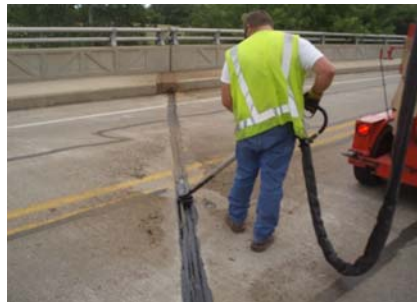
2011 Crack Sealing Program
