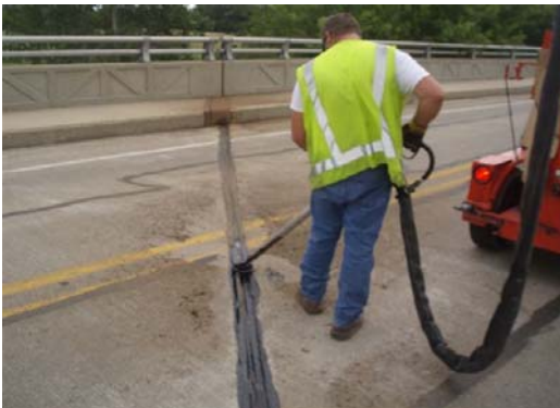
2012 Crack Sealing Program
