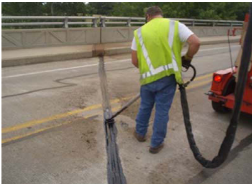
2013 Crack Sealing Program
