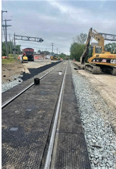
DIXIE HWY RR CROSSING
