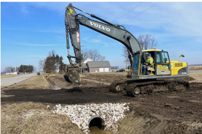
Corunna Rd (Ditch & Johnstone) - Chesaning Twp Ditching & Culvert Replacement
